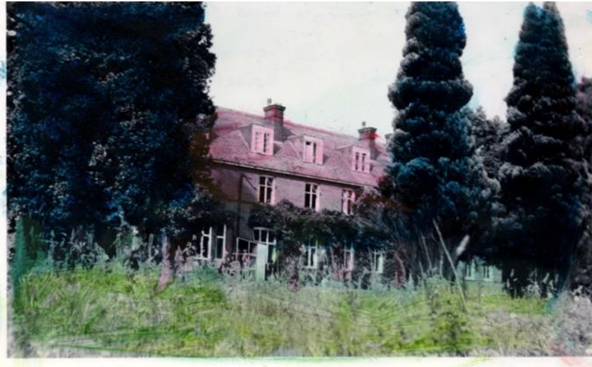
St Mary's Hill seemingly just prior to demolition
